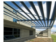
Reno ANGB (shading in building design)
