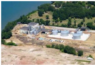
Biodiesel Manufacturing Facility Confidential Client, Confidential Location
